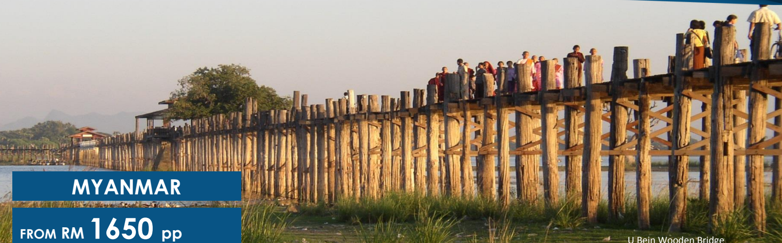
U Bein Wooden Bridge
